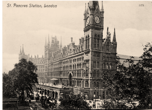
Figure 3: St. Pancras Railway Station Building
